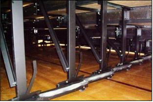
An extruded aluminum H clip is placed between the sections. Deck boards are finished with a layer of high density polyethylene plastic (panel am) .025 - .030 thick.
